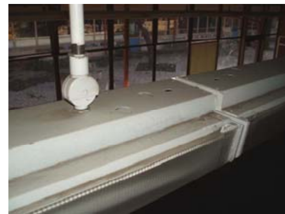
Figure 11 – Typical unidirectional swivel used on the bottom of the pendant stem in Havens ES. This detail allows stem rotation in one direction.
