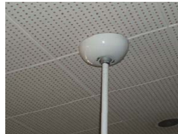
Figure 10 – Typical ball and swivel top connection of pendant fluorescent light fixture in Havens ES classrooms.
