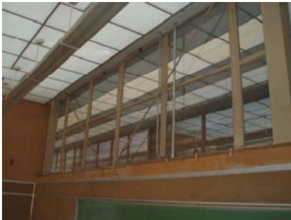
Figure 2 – Interior of a classroom wing showing rod bracing adjacent a corridor. Four bays of bracing, two on each side of the corridor, provide the longitudinal seismic resistance. Note the overhead glass in the corridor wall.
