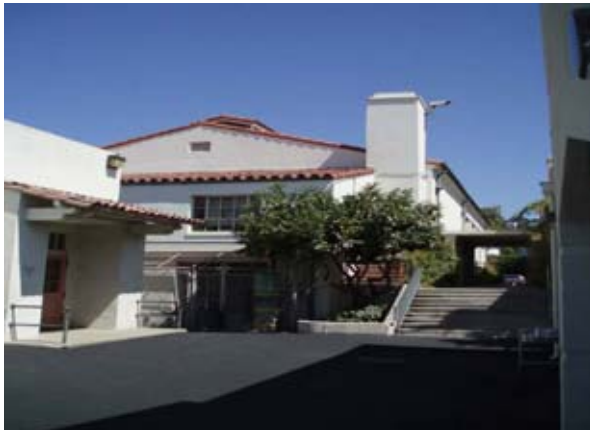
Figure 8 - Rear of Building C showing the concrete portion of the building. The chimney shown has reinforced concrete construction.
