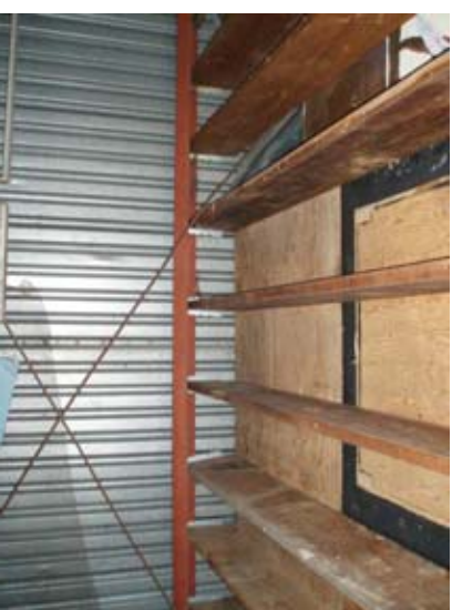
Figure 13 – An ad hoc mezzanine was installed in S/E corner of the prefab building. Materials on it are unrestrained and can fall off.
