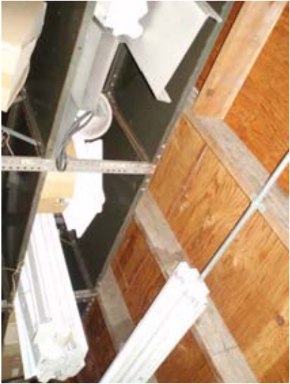
Figure 15 – The west mezzanine is partially supported on the tops of steel shelving.
