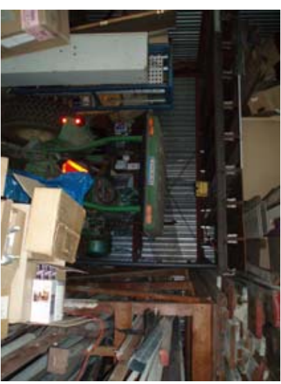
Figure 13 – An ad hoc mezzanine was installed in S/E corner of the prefab building. Materials on it are unrestrained and can fall off.
