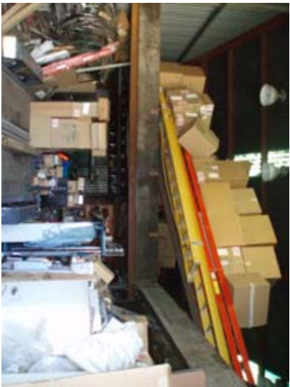
Figure 11 – Boxes are stored on a ladder placed horizontally. These constitute a falling hazard, and the storage arrangement does not meet ASCE 31 requirements.
