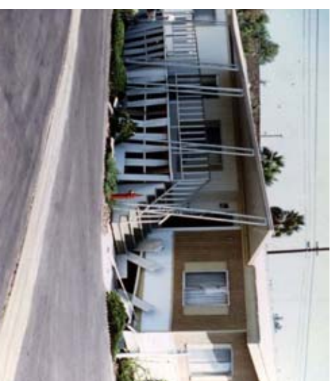
Figure 8 – An example of a trailer (mobile home) that has fallen off its supports.
