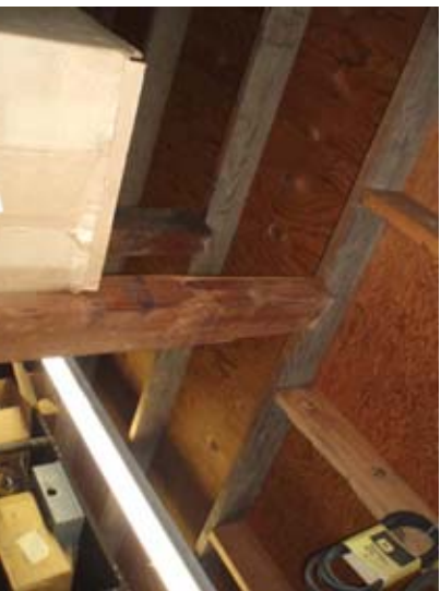
Figure 15 – The west mezzanine is partially supported on the tops of steel shelving.
